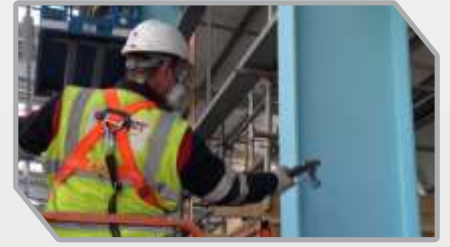
Fire Protection Coating
