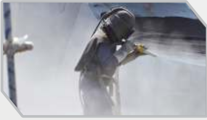
Surface Preparation Sandblasting
